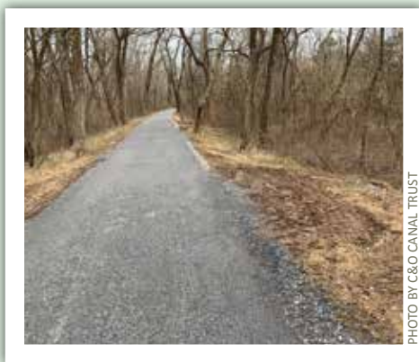
The new towpath surface is crushed stone dust, the same material that is used on the Great Allegheny Passage (GAP).
