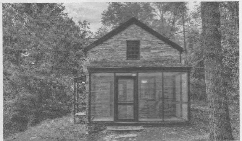
Lockhouse 10, in Cabin John, Maryland, features a screened-in porch and is nestled in the trees above the canal and towpath.
