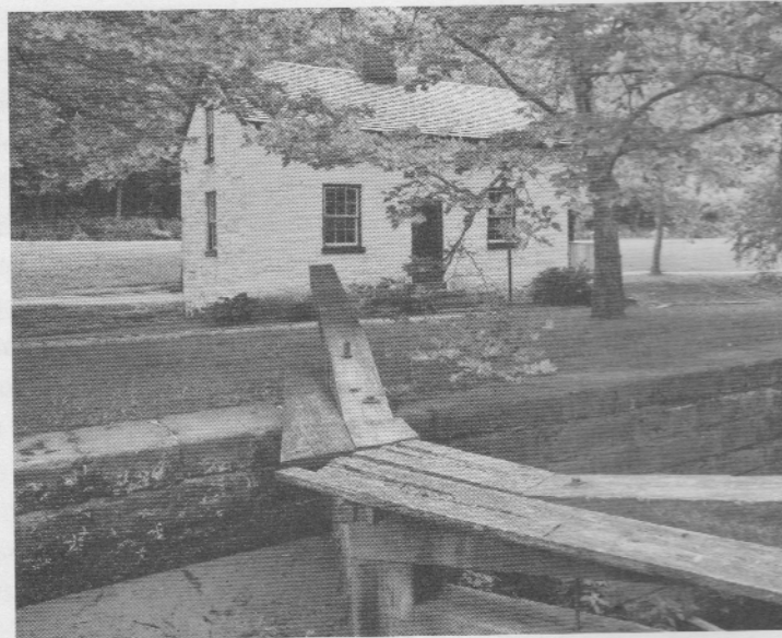
Lockhouse 6 is perched along Lock 6 in Brookmont, Maryland, at mile marker 5.4. Photographs courtesy of the C&O Canal National Historical Park, the C&O Canal Trust and Heidi Glatfelter.
