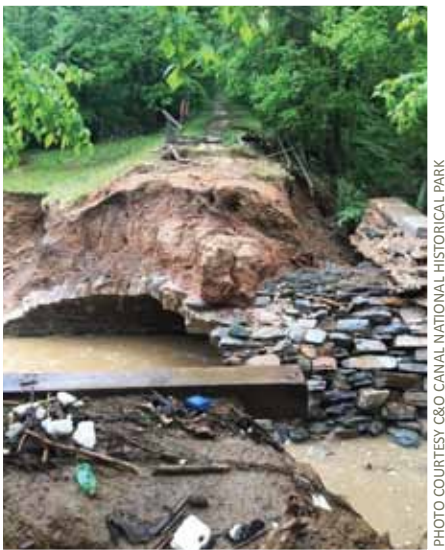
The towpath washed out at culvert 82 near Brunswick due to flood waters.
