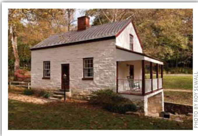
Lockhouse 6 stands in Brookmont and was one of the first three lockhouses to open in 2009.
